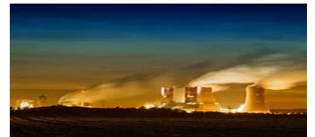
Oil & Gas Engineering
