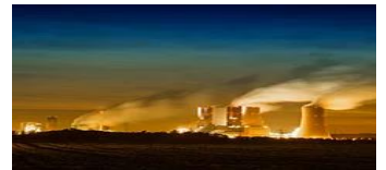
Oil & Gas Engineering
