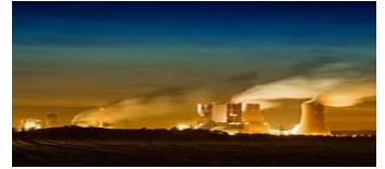
Oil & Gas Engineering
