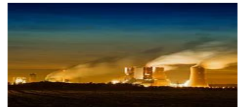
Oil & Gas Engineering
